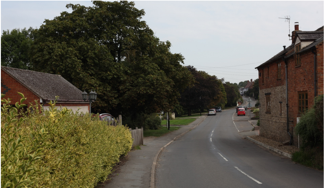
Figure EDP 4.2: Street character to site (left, out of picture) with frontage of mature trees
