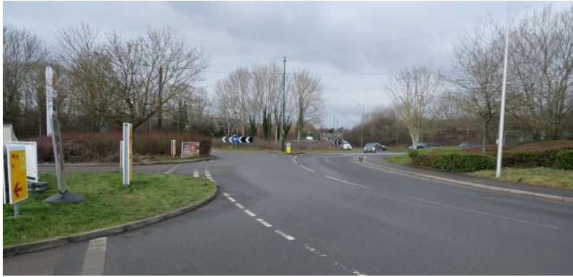
View north-west towards the existing roundabout on the A423
