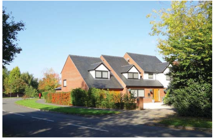
Improved property on Dencer Drive
