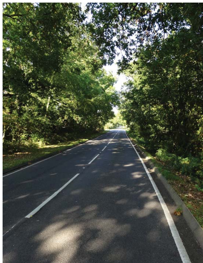
New pedestrian crossings required along Glasshouse Lane
