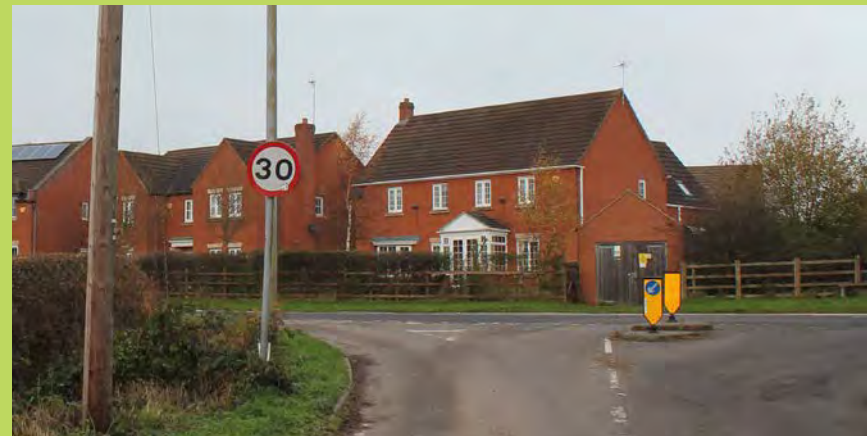
Substation on Westwood Heath Road
