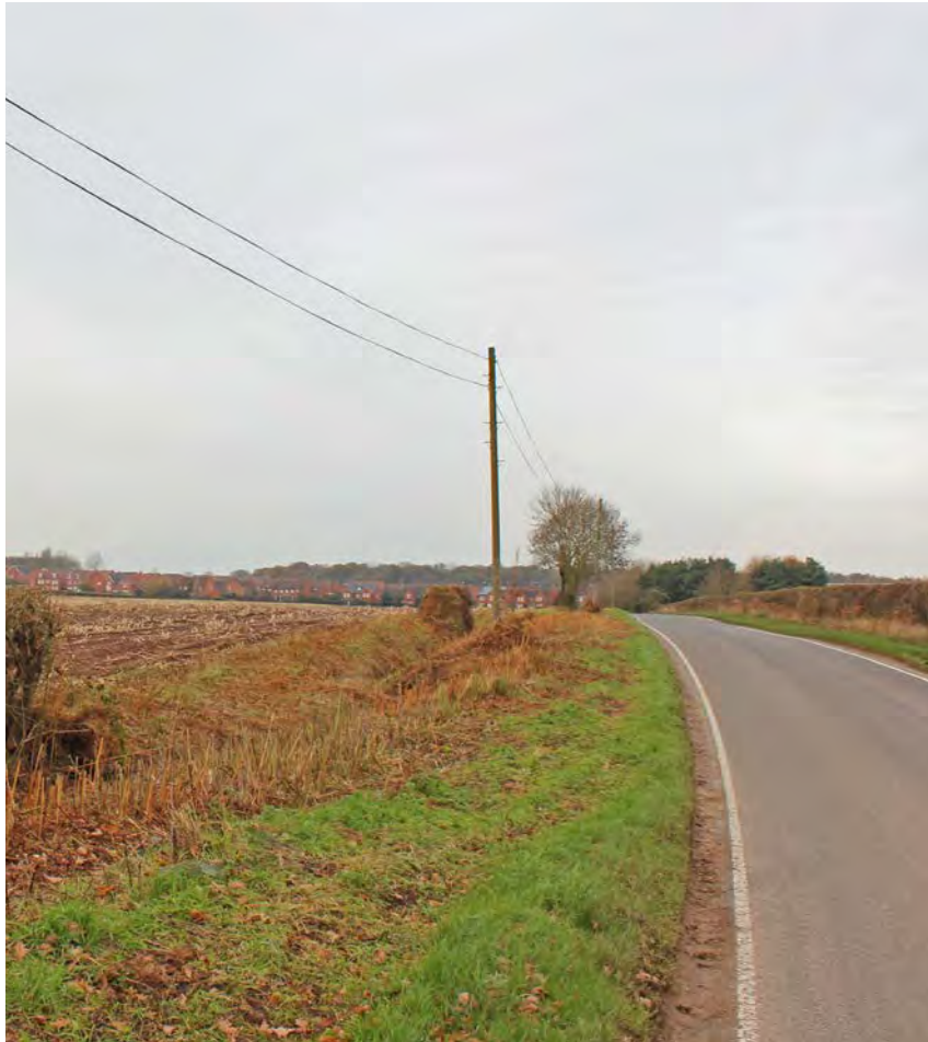
View along Bockendon Road
