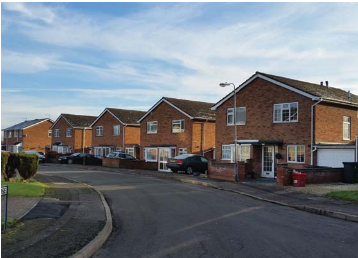
1970s semi-detached properties on Langdale Close
