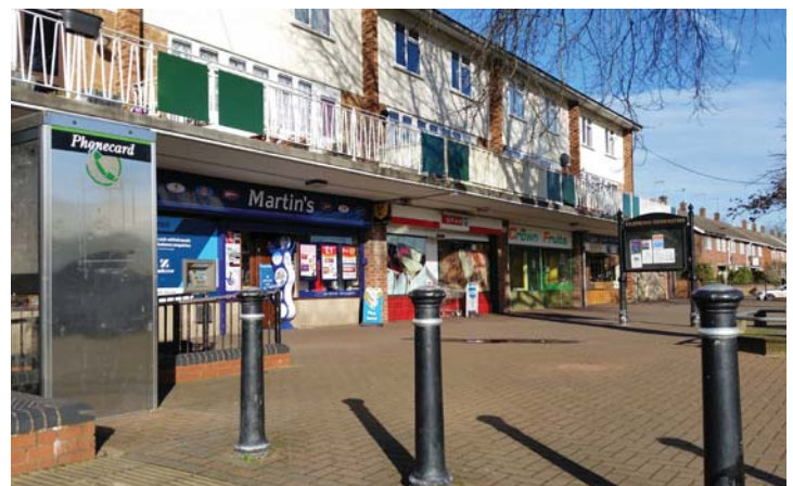
Crown Way Local Centre having accommodation above
