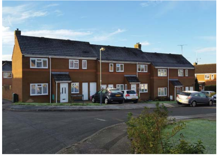
Late 20th century terraced accommodation along Wackrill Avenue
