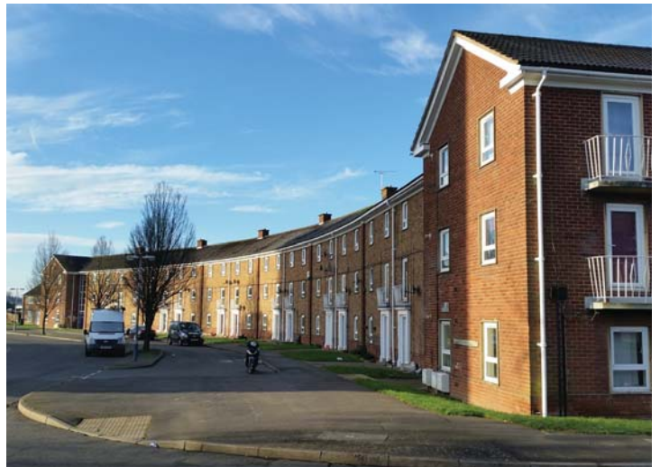
Strong block form/focal building on Newland Road
