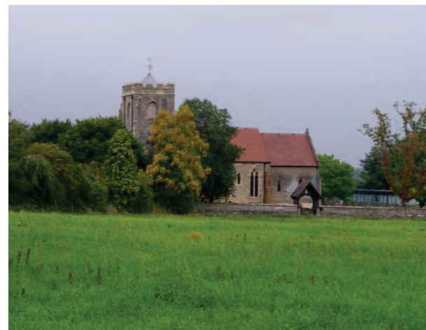
Figure 13: View looking north from Southam Road towards the Grade II Listed Parish Church of St Nicholas.
