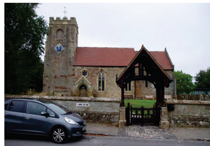
Figure 18: South façade of Grade II Listed Parish Church of St Nicholas with Grade II Listed stone boundary wall and timber Lychgate.
