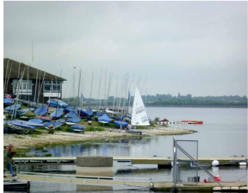
Draycote Reservoir provides local drinking water and is a valuable recreational and biodiversity resource.
