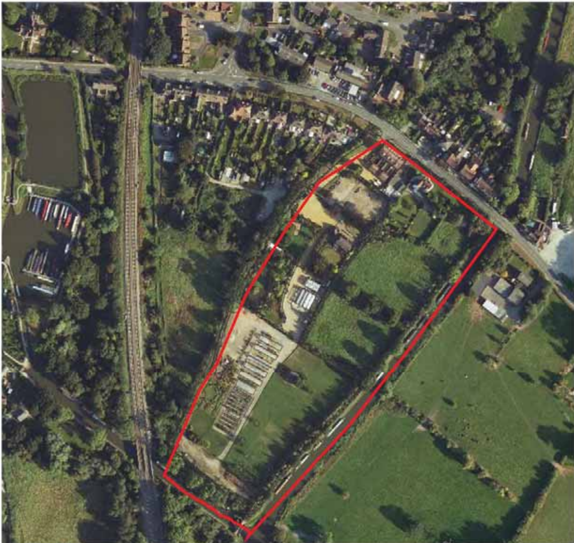
Figure 2: Development Site Photograph with Topographic info overlaid
