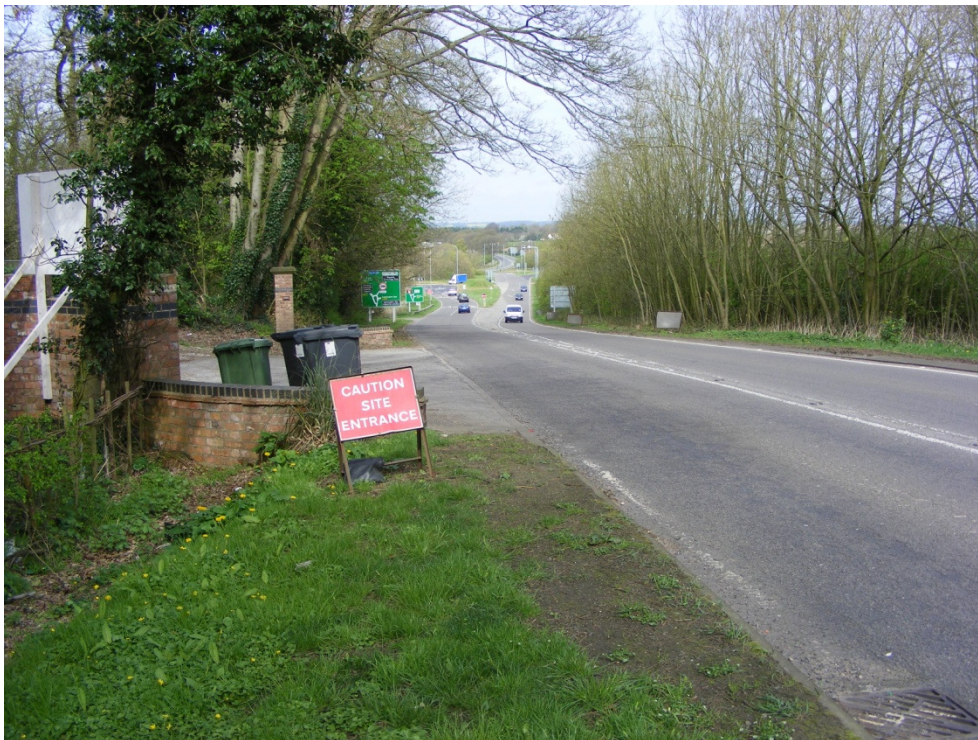
Figure 8 The A452 Half Moon Plantation Access looking towards Greys Mallory Roundabout
