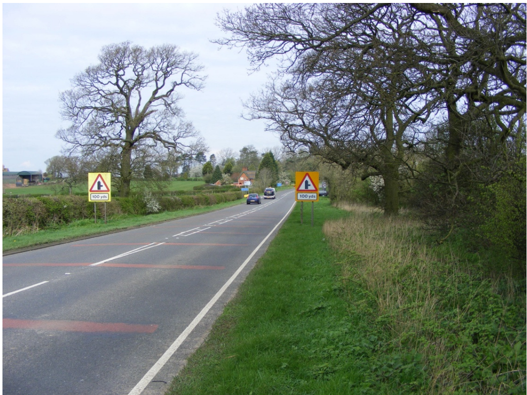
Figure 2 Southern approach to the A452/Mallory Road Junction showing the yellow bar line traffic calming
