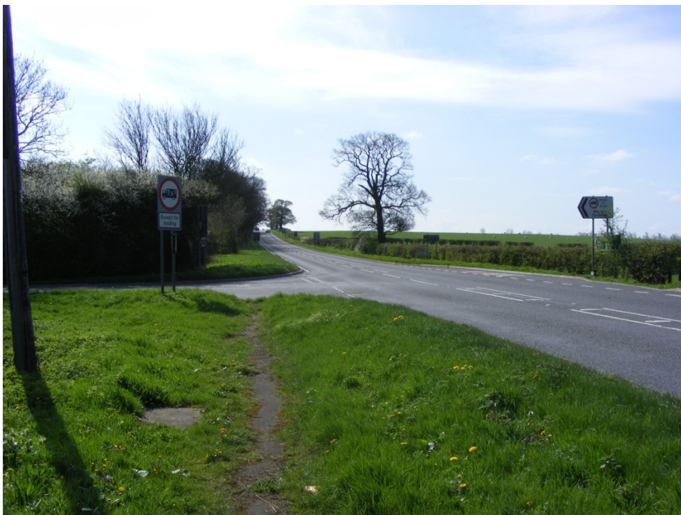
Figure 6 The A452 Banbury Road/Mallory Road Junction looking towards Hill Farm
