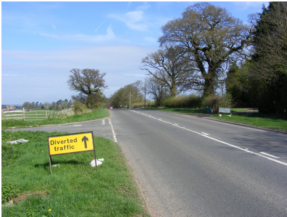
Figure 5 The A452 Banbury Road/Hareway Lane Junction
