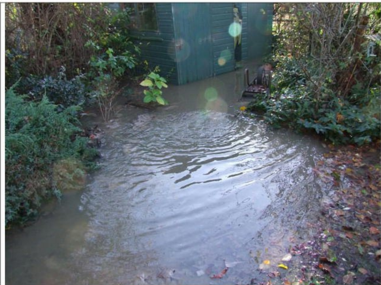
Garden at Daly Avenue flooded with raw sewage from surcharging manhole – December 2012
